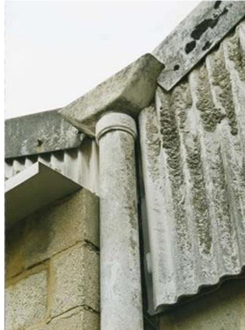
Asbestos cement downpipe, hopper and profile sheet
