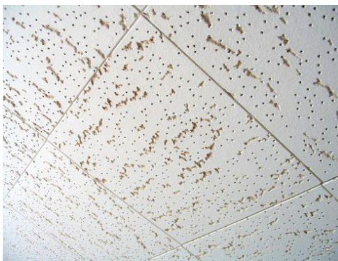
Asbestos containing ceiling tiles
